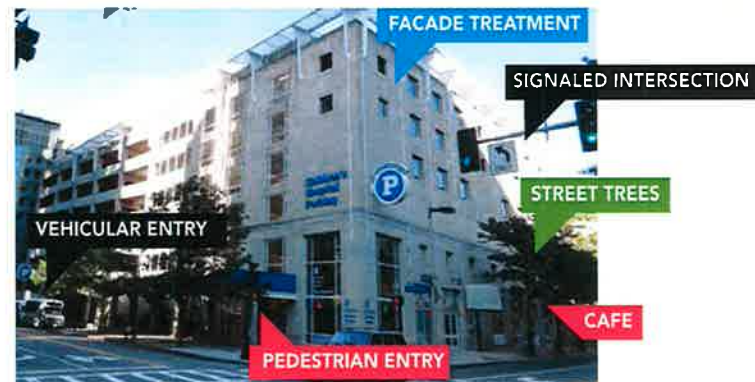
Example of parking structure with active ground floor along a principal street, including a cafe. The façade treatment on the main street conceals views of automobiles from the main street, enabling the structure to blend in with its surroundings.
